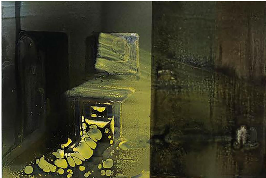
Though boarded up and without electricity or running water, the Barrow family's gas station still stood at 1221 Singleton Boulevard (formerly Eagle Ford Road) until April of this year. Brief glimpses inside, through cracks in the exterior and a crescent-shaped gap in the front door, provided the basis for her paintings. Michelle Mackey
